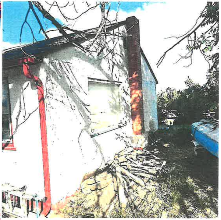
View East from SW corner of garage
